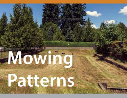
Alternate mowing patterns and keep off wet soils to prevent ruts from forming, which can lead to channeling and costly overhauls.
