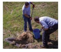
**Step 3:** Use a shovel, post-hole digger or wet-dry vacuum to remove sediment.
