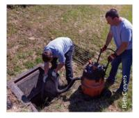
**Step 2:** Remove grate using proper lifting technique and set aside. CAUTION - grate is heavy.
