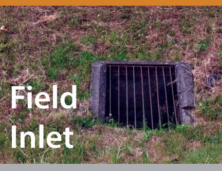
Maintaining your field inlet, or grated inlet, should be done periodically and can usually be performed with common tools.
