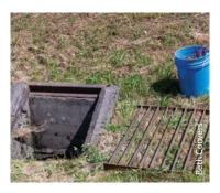
**Step 4:** Reinstall grate, bag sediment and dispose in the trash. DO NOT put in yard waste cart or compost.
