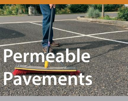
Permeable pavements need periodic maintenance, such as sweeping and pressure washing without soap, to function properly.
