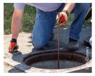
**Step 4:** Reinstall cover. Dispose of material in regular trash. CAUTION: sediment may be contaminated - DO NOT put in yard debris cart or compost.
