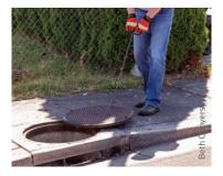
**Step 3:** If sediment is 60% or more of the sump depth, remove sediment and bag it for disposal.
