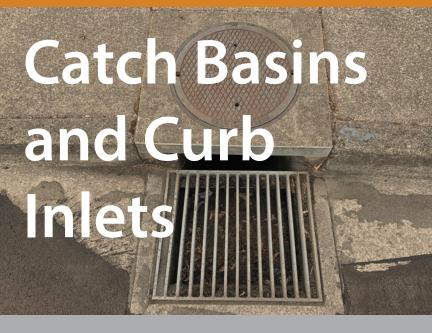
Catch basins and curb inlets must be cleaned periodically to effectively trap sediment and allow stormwater to flow into your facility.
