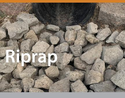
Maintain riprap during summer months when the weather is dry. Regular maintenance is possible with common tools, but bigger jobs may require an excavator.
