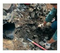
**Step 4:** Replace riprap so multiple layers cover native soil. Dispose of sediment in trash.
