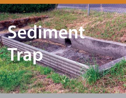
Make sure sediment traps are maintained annually to keep your stormwater facility functioning properly.
