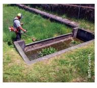
**Step 2:** Use a shovel to scrape dirt and debris off the bottom of the sediment trap.
