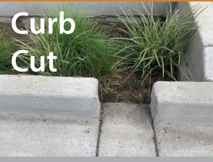
Use common tools to clear sediment and debris from curb cuts to prevent puddling and allow stormwater to enter your facility for treatment.
